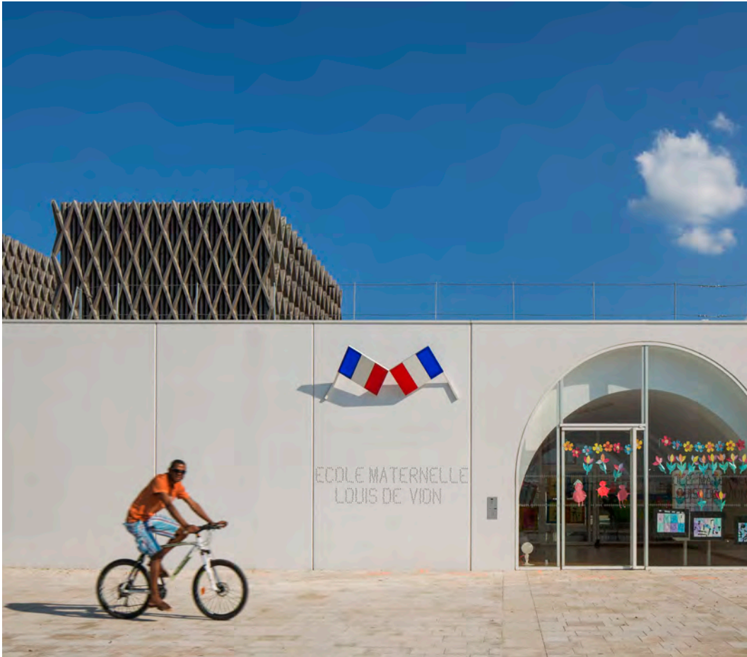
© AAVP – Atelier Architecture Vincent Parreira – Photographie Luc Boegly
